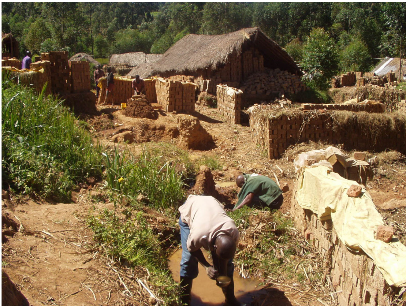
Figure 1 Brick-making site in the Kenyan highlands. Assessments of the shallow pools dug by brick-makers is taking place in the foreground as brick makers continue to excavate soil, combine the soil with water, mould the resulting mud into bricks, and then left to dry before firing.
